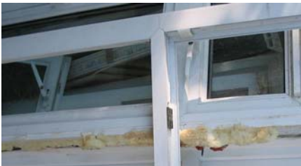
Figure 16. Foam contamination
