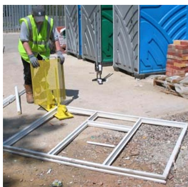
Figure 12. Corner cutter trialled for volume reduction
