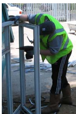
Figure 13. Use of cordless power tools to aid deconstruction onsite
